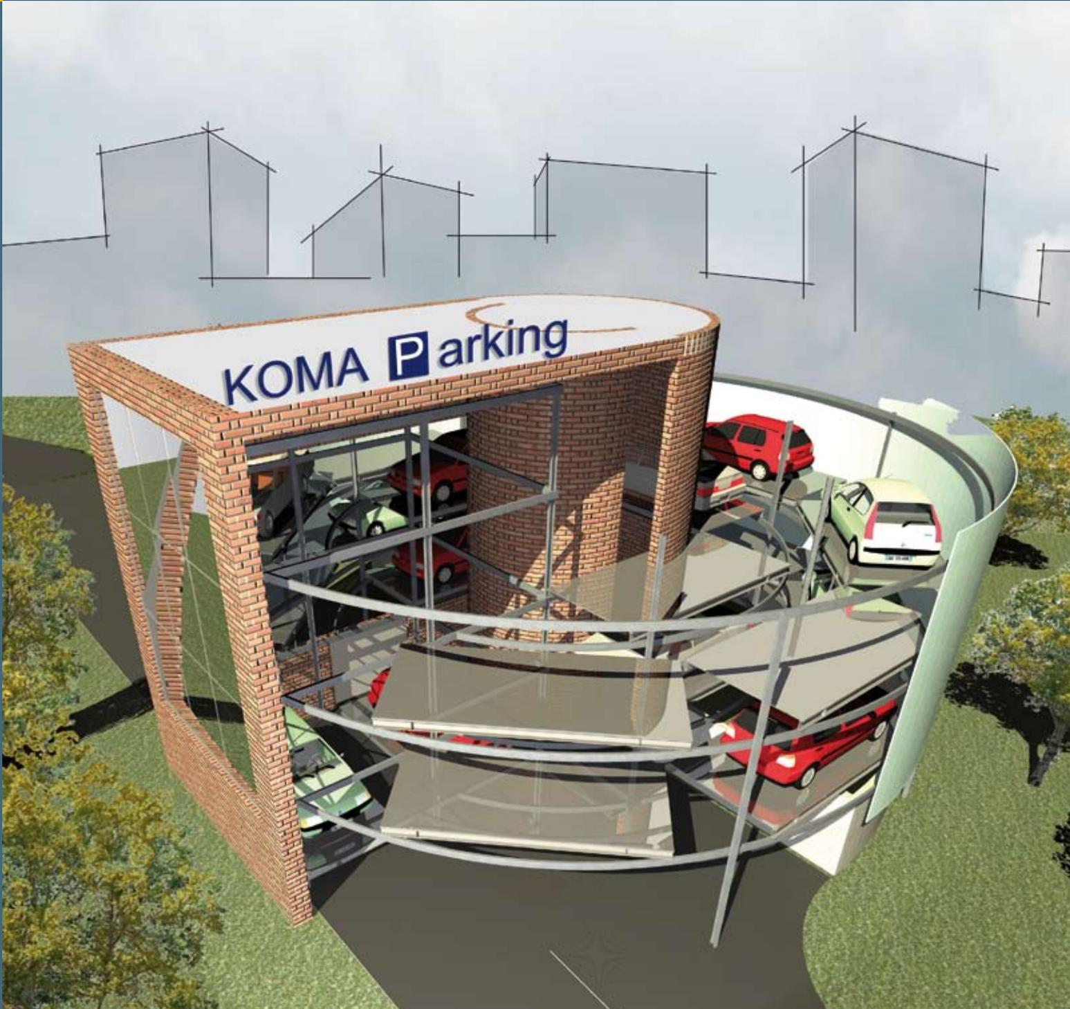
An automatic system for independent parking making a full use of available parking space by placing cars onto pallets arranged circularly in particular annular rings and on top of one another. For indoor application only. Available varieties for use above ground, under ground and combined. It is also suitable for subscriber parking and park timing.
